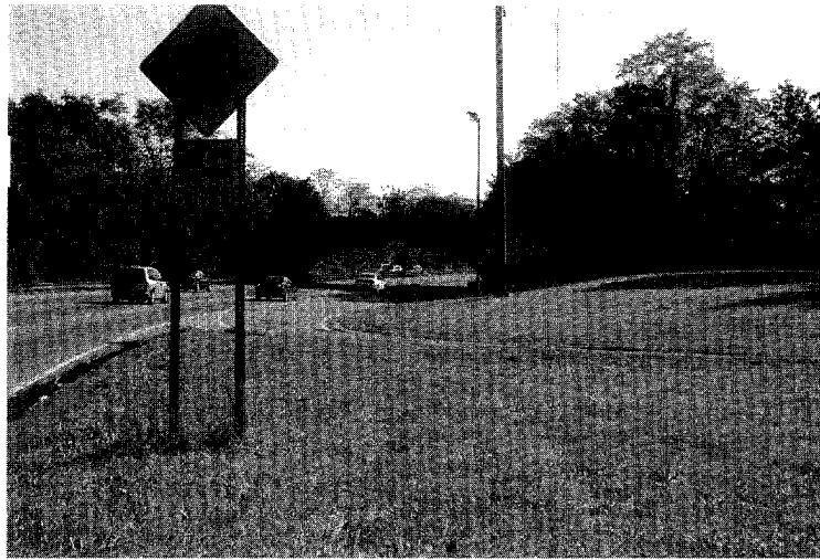
Figure 3.12: A Sight Restriction on a Horizontal Curve
