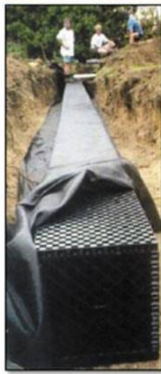
Step 3: Cover with Atlantis Hydronet & backfill.
