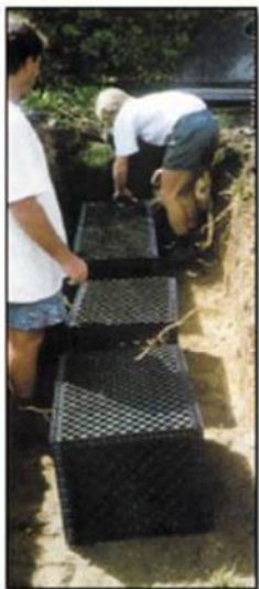
Step 1: Lay tanks in trench
